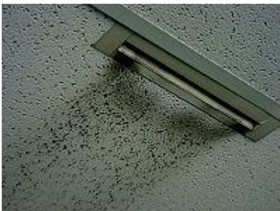
Indoor air pollutant particles (diesel fumes and soot type), left on the ceiling around an air inlet.
